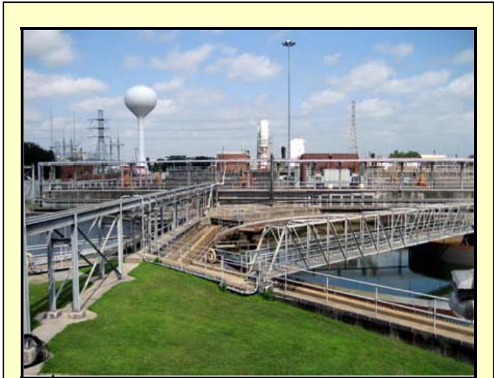
69 th Street Wastewater Plant May 21, 2008 Photo by Susan Smyer
